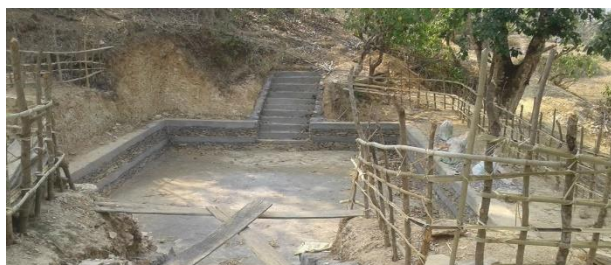
Plate 1: Recharge Ponds for spring Revival included in design estimates of Bohochhap Solar Lift DWSS Ghiringsundhara VDC, Tanahun
