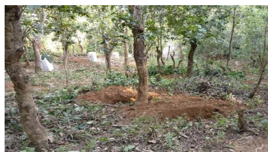
Plate 2: Recharge pits for spring Revival included in design estimates of Bohochhap Solar Lift DWSS Ghiringsundhara VDC, Tanahun
