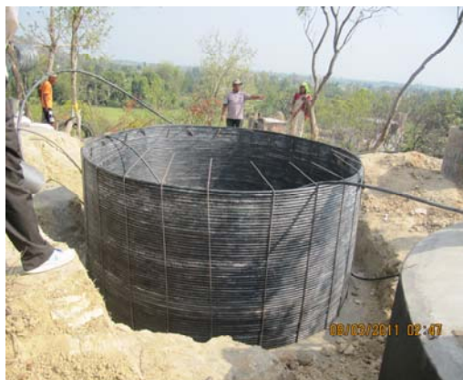
Elevated Tank, Sorauli, Rupandehi
