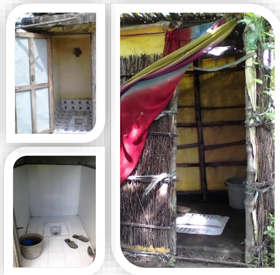
Photo: There are many options for constructing a toilet that is safe and hygienic to use with dignity.
