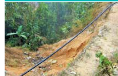
Exposed pipeline is a risk for scheme functionality.
