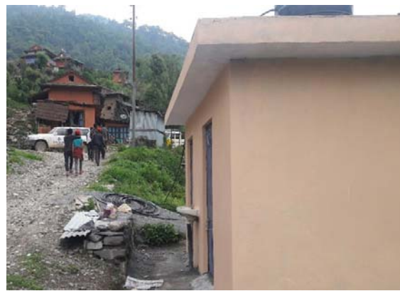
Figure 1: Public toilet in Bharse VDC
