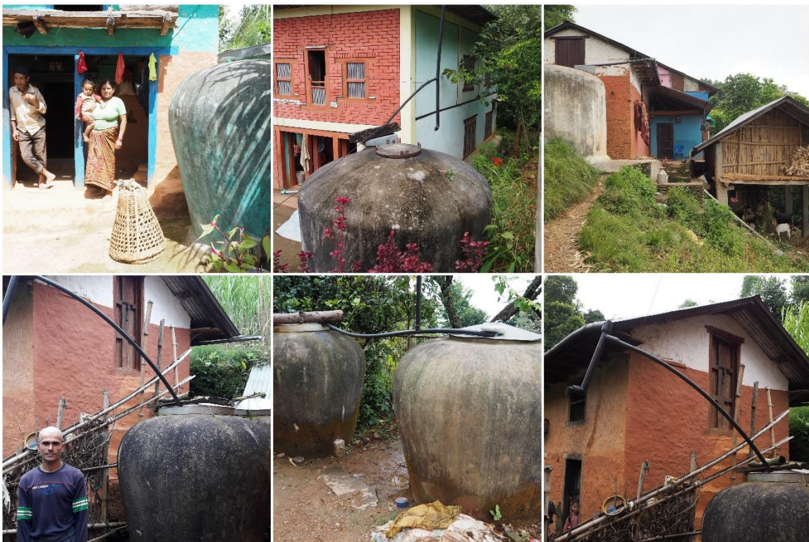
Photo 1. Rainwater harvesting jars after more than a decade in Gulmi district
