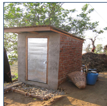
Figure 2: Latrine with brick
