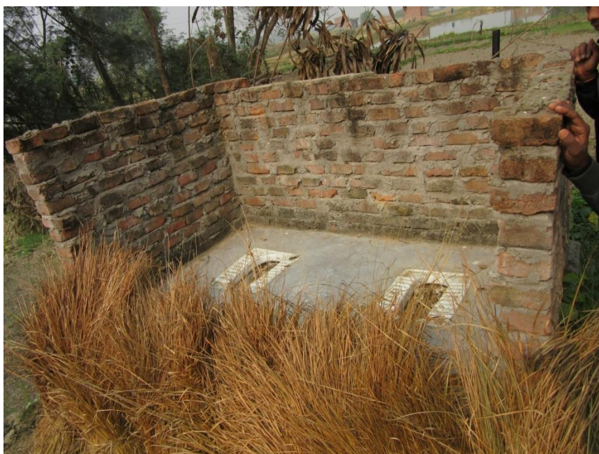
Photo 3 Subsidized toilet with incomplete superstructure, Rupandehi
