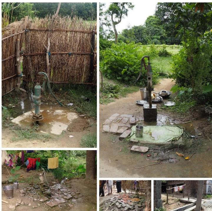
Environmental sanitation counts! For many Tarai communities, drainage causes critical sanitation problem. Poor drainage as in these photos contaminate the shallow tube wells, and breed mosquitoes.
